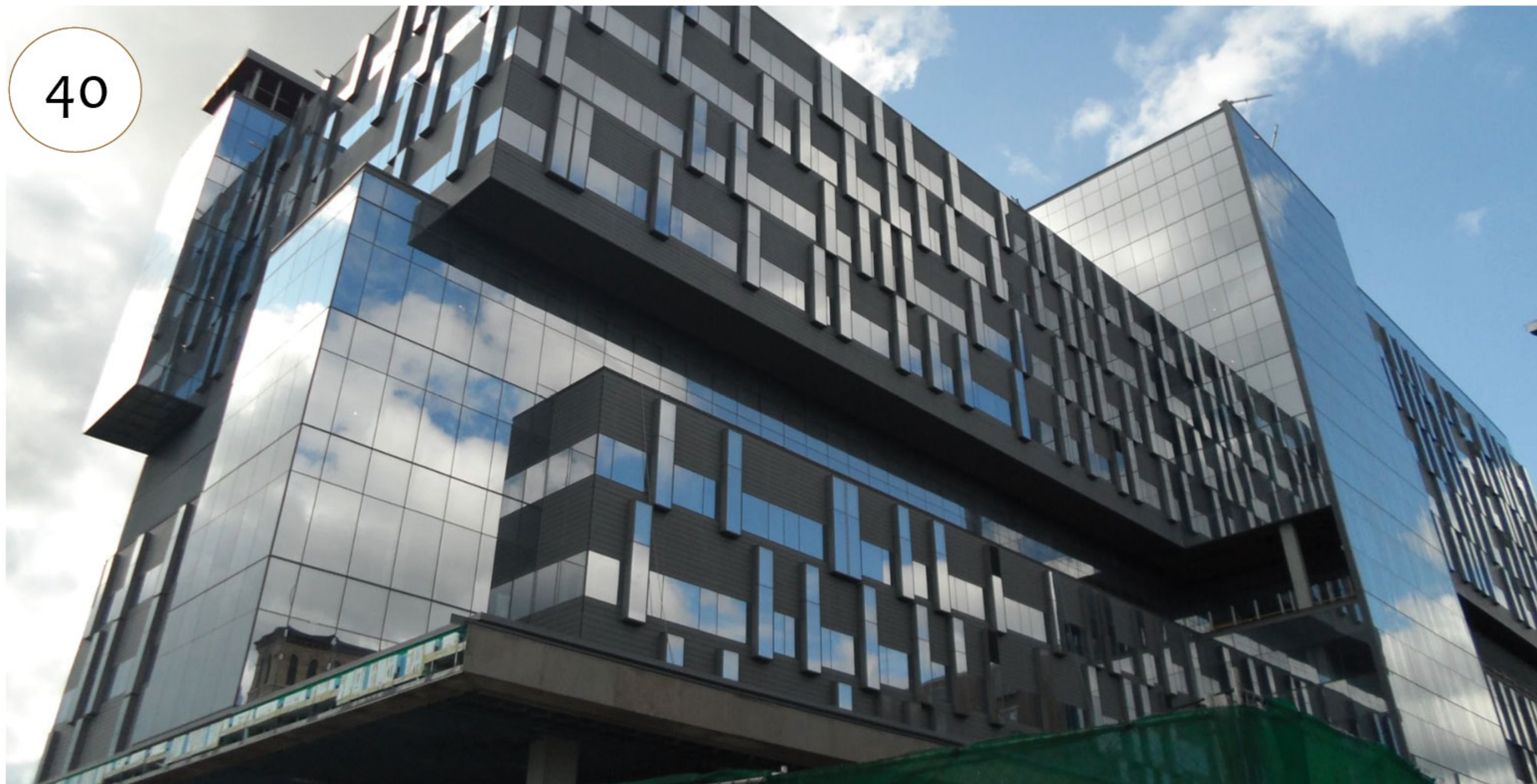
BRIDGEPOINT HOSPITAL [BASS INSTALLATIONS]
